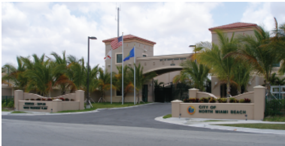
Figure 1: Newly Improved Norwood-Oeffler Water Treatment Plant
