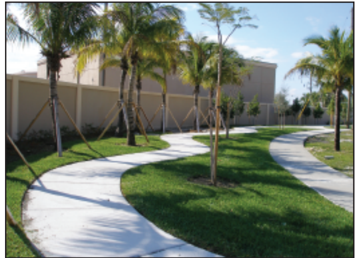
Figure 8: Concrete Panel Screen Wall
