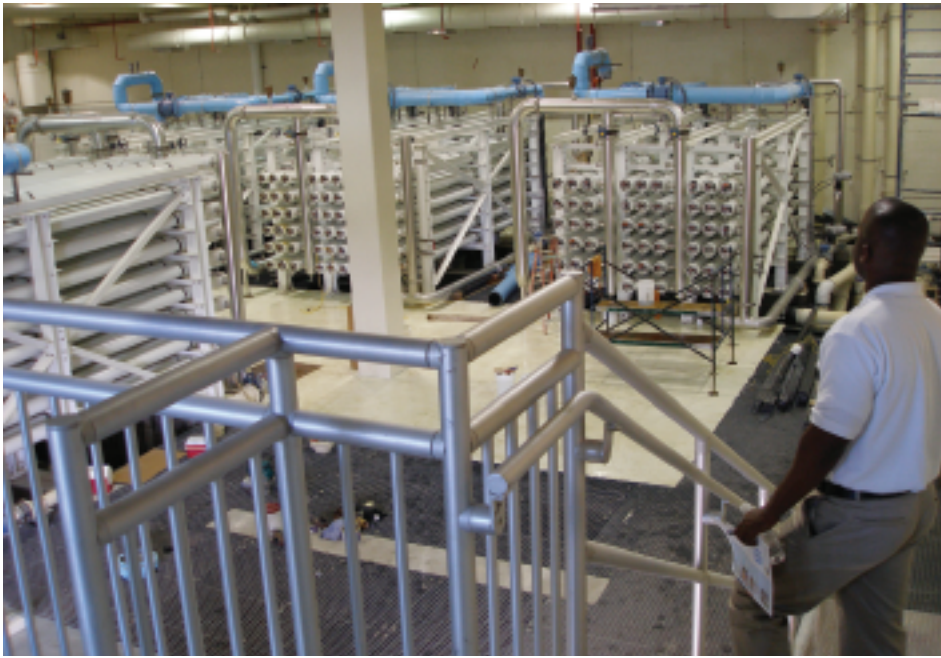
Figure 2: New 31,500 Square-Foot Norwood Water Treatment Plant Process Building
